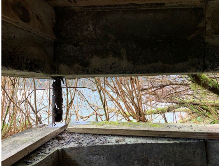
Figure 4 – Deteriorated Steel Pipe Supports
