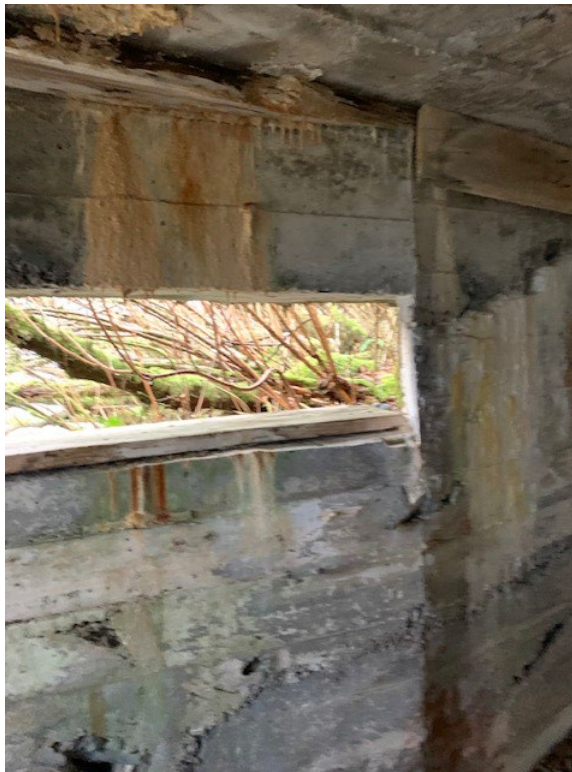
Figure 1 - Colored Efflorescence on Walls and Roof
