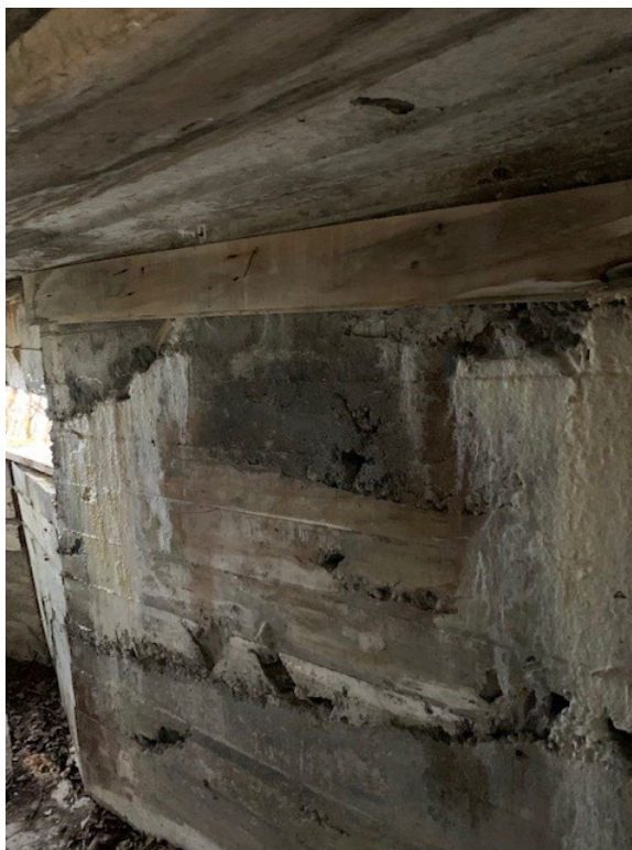
Figure 2 – Pockets in Wall Concrete
